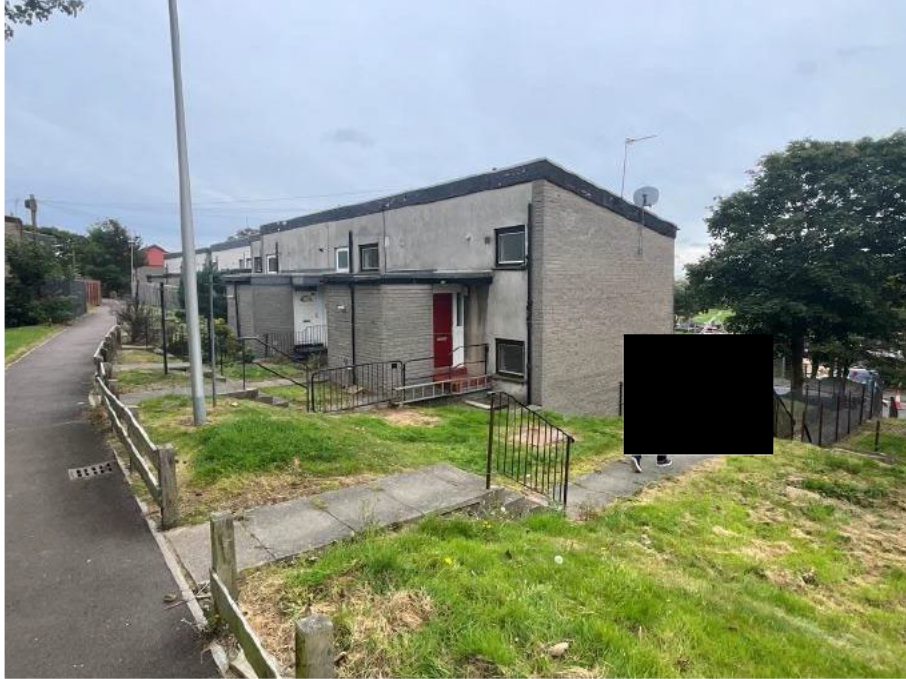
Figure 6: Original 'flat' roof system
