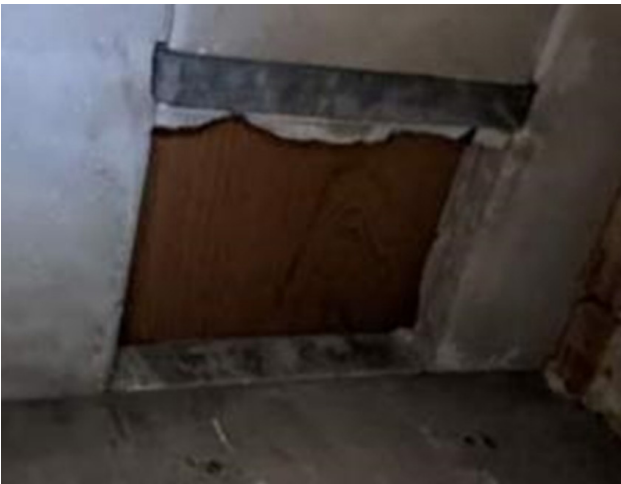
Figure 4 – Photo of hangers
