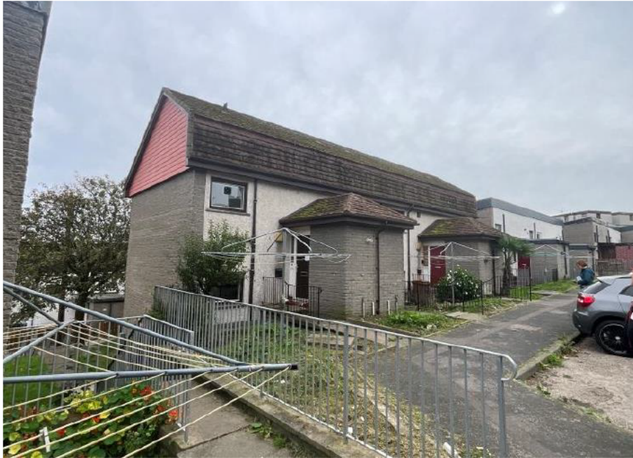
Figure 10: Refurbished mansard roof system
